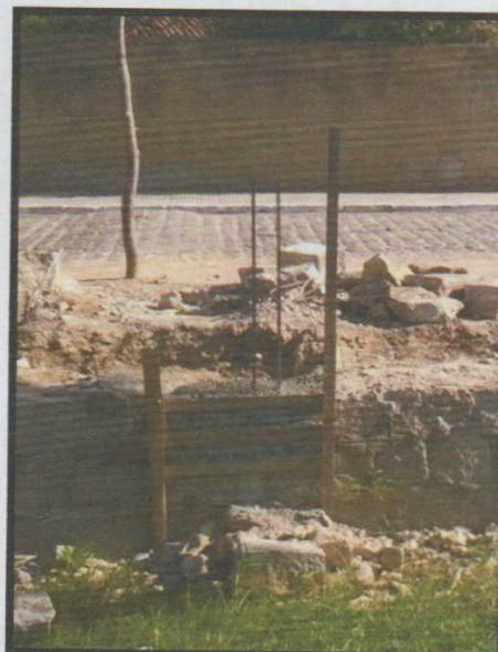
Figura 16: Sapata concretada
